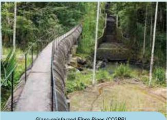
Glass-reinforced Fibre Pipes (CCGRP)
