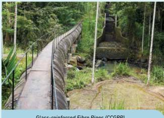
Glass-reinforced Fibre Pipes (CCGRP)
